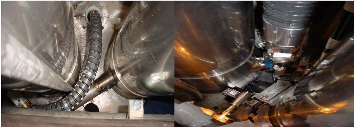
Ringhals Inspection Arm
