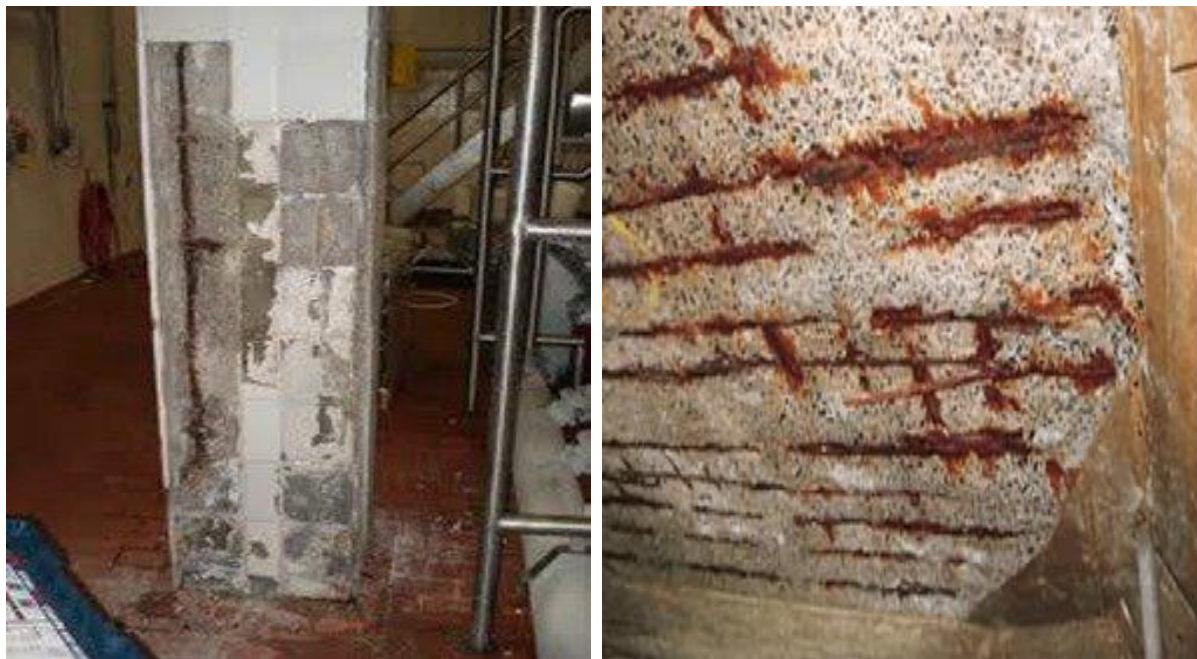
Chemical attack on concrete columns
