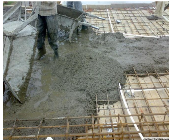
Placing of concrete
