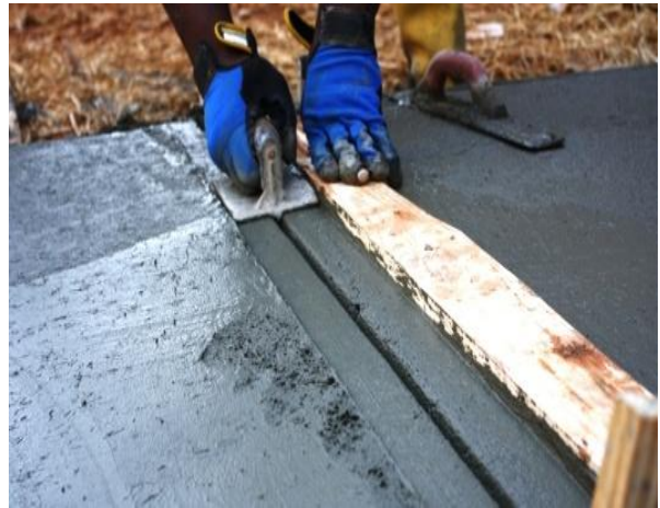
Groover (Grooving for joints)
