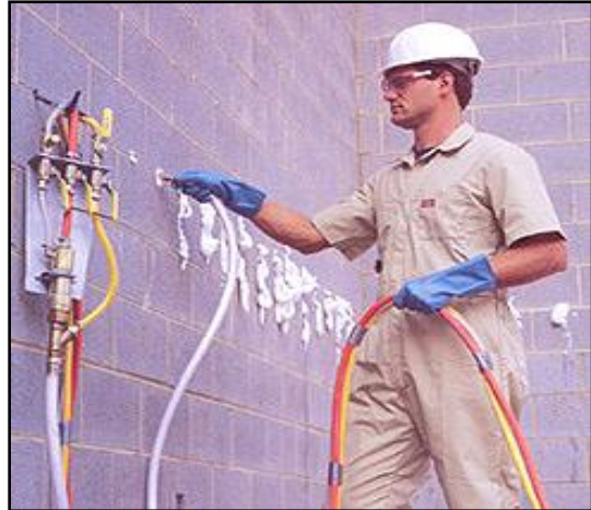
Concrete block insulation method
