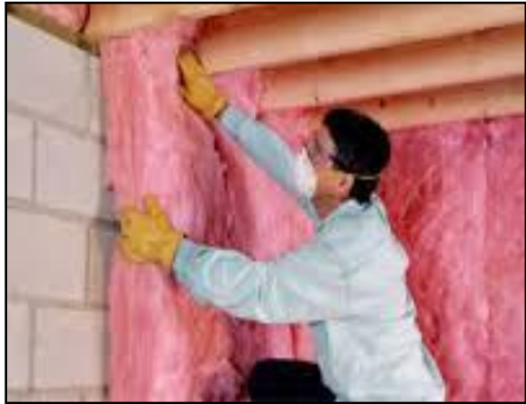
Blanket batts and rolls insulation method
