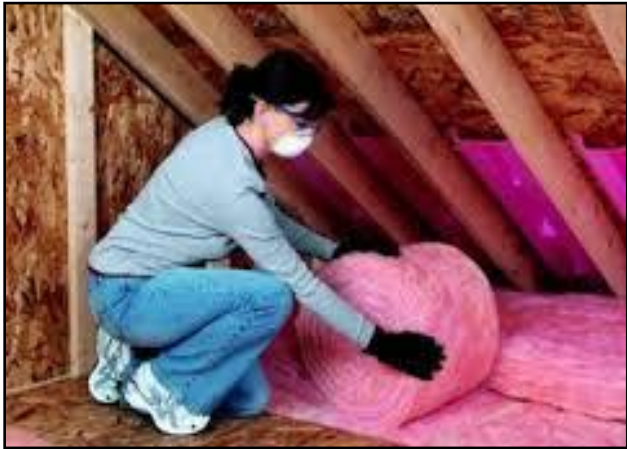
Blanket batts and rolls insulation method
